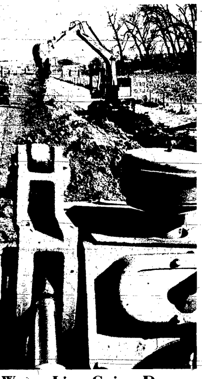
Water Line Going Down. WORKMEN for a Honey Creek, Ia., construction firm were last week putting down a water line east of Wayne. Work on the project began Monday morning on the south side of Highway 35 for the line which will lead to the city's industrial site just east of town. The city council approved the approximate $31,000 project during a recent council meeting.
